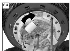
Place light kit over screws and twist direction of arrow into place. Then tighten all 3 screws securely.
